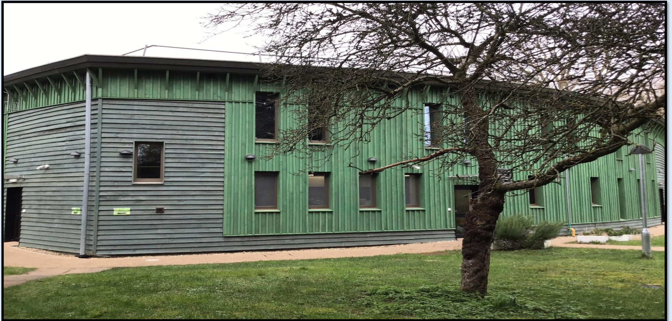
The Ark (Dining room, meeting rooms and accommodation)
